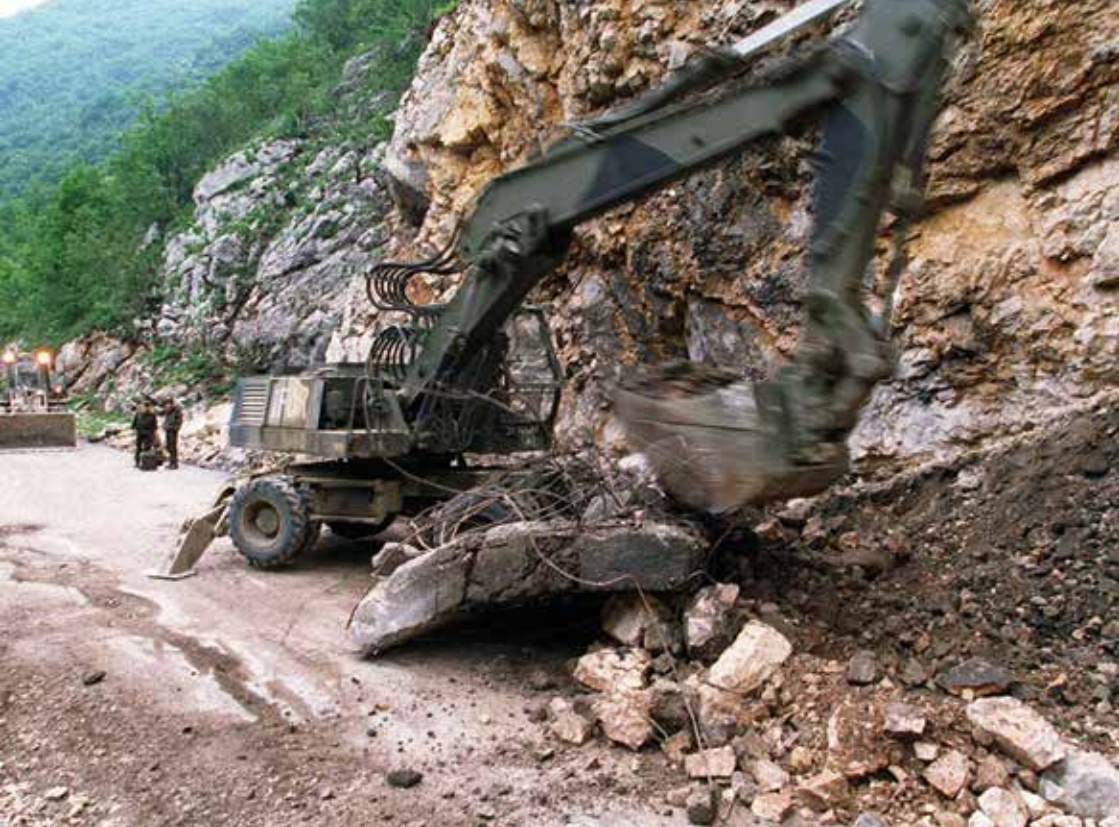
Picture shows a Royal Engineer excavator helping to remove rubble from the mouth of the Cloutman Tunnel near Jajce, Bosnia. It took British Royal Engineers working in Bosnia just two days to clear the mouth of rubble and debris on a route which, when opened, will cut miles off vital journeys for local residents. Photo: Mark Owens, Crown Copyright
