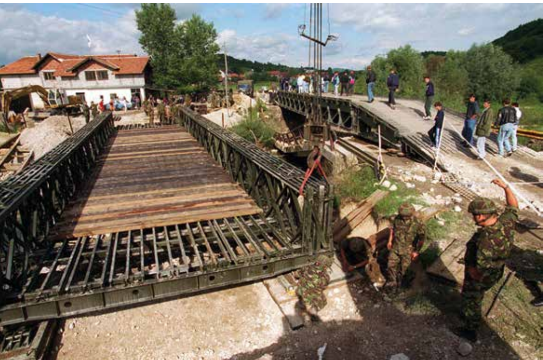
Local population view the construction of a Bailey bridge at Fajtoy, near Sanski Most, which when finished will allow buses to travel through to their village. The bridge was constructed by 3 Armoured Squadron, 22 Regiment Royal Engineers. Photo: Captain Kevin Harvey, Crown Copyright
