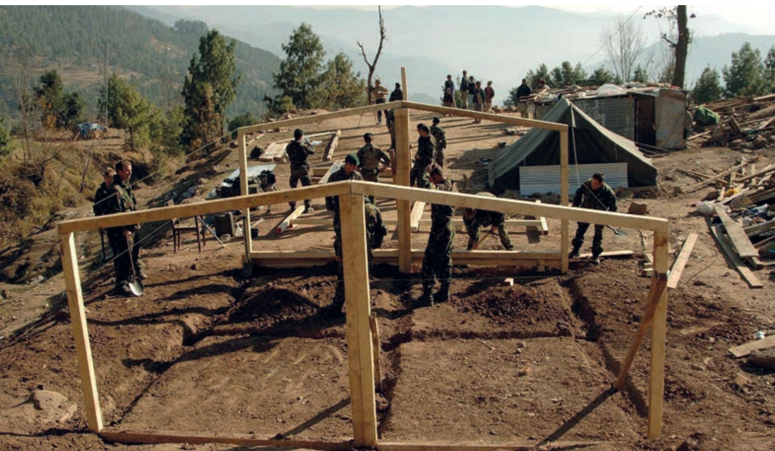
Eighty-six engineers from 59 Independent Squadron Royal Engineers and Royal Marine engineers from Plymouth built shelters in Bagh District, Kashmir, as part of the United Kingdom's Department for International Development, programme of aid to Pakistan after the earthquake on 8 Oct 2005. The troops travelled up to remote mountain villages up to 7,500 ft to construct shelters for medical and school facilities. Photo: Phot Ian Richards, Crown Copyright
