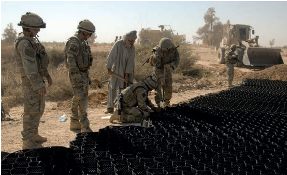
Members of 9 Squadron Royal Engineers and 23 Engineer Regiment are pictured building a road with the assistance of local Afghans. The road links to a bridge across the Loy Mandeh Wadi. The bridge will then be rebuilt to enable access for heavy goods vehicles, opening supply routes across the area. Photo: Corporal Mark Webster, Crown Copyright
