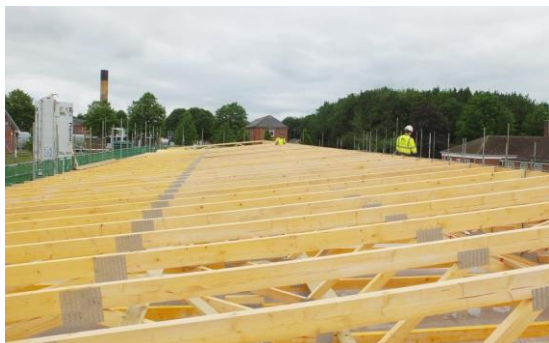
Construction works at Bulford
