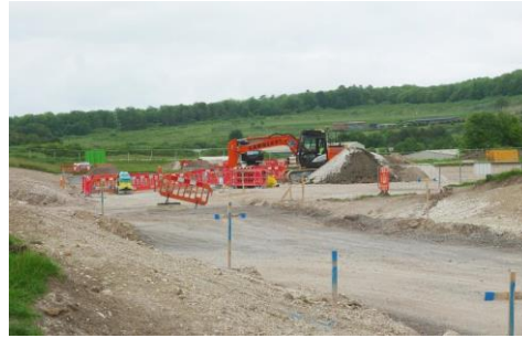
Construction works at Tidworth for Mess and SLA
